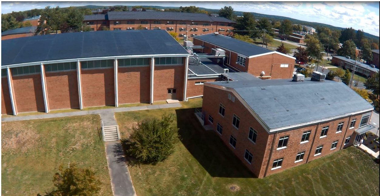
Above: LEWA Devens Bioprocess Systems Manufacturing Complex, Devens, MA USA
